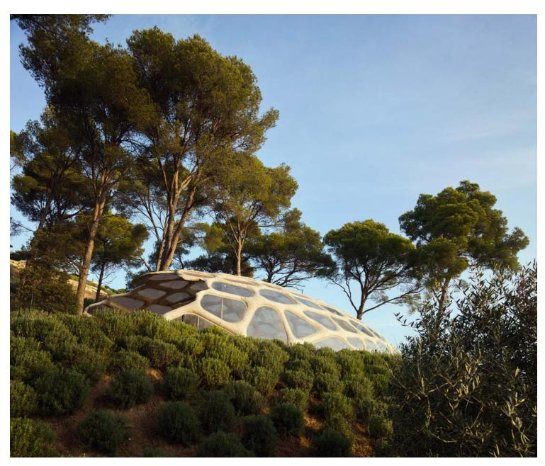
The pavilion structure, developed through the creation of prototypes, is derived from an inflatable framework, injected with lightweight and ecological smart concrete, resulting in an organic form inspired by the pine trees all around.
