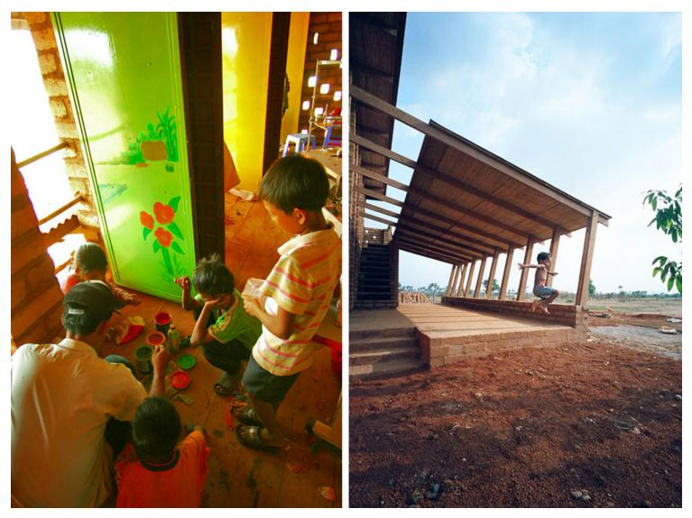
The school building is made out of local materials and build using the local workforce. The aim was to encourage the community to make the most out of the materials that are easily available. The building budget was extremely low and the materials were scarce, so the beautiful red soil was utilized as the main construction material in the form of sundried soil blocks.
