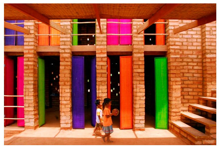
The soil block walls are laid out with small holes, so that indirect sunlight and gentle wind come in to cool the spaces. The community area is open, providing comfortable shade from the sun.
