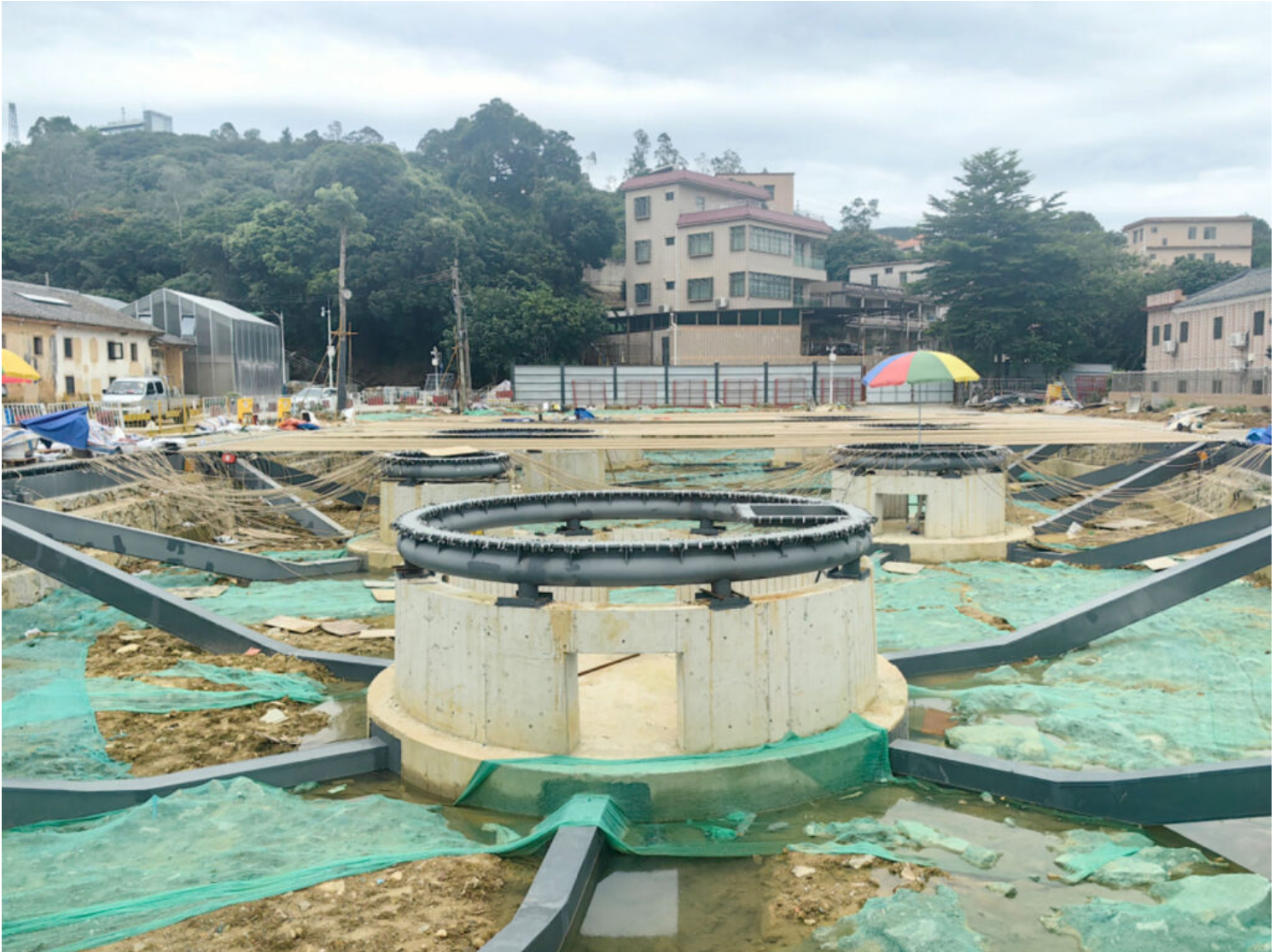
"Soft Square" under construction © Zhu Xiaodi
