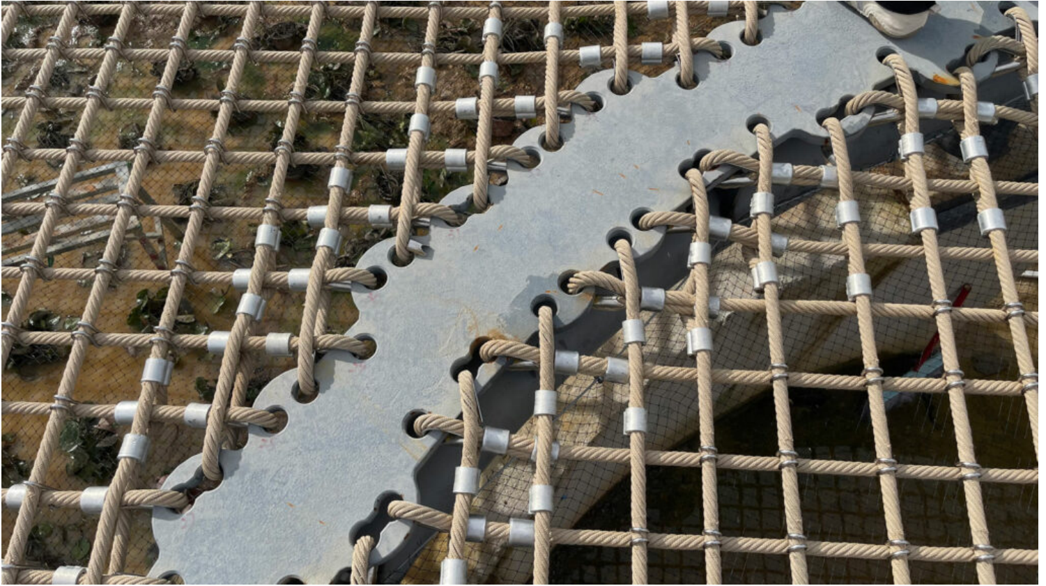
Circular supportive structure of the rope net installation © Zhu Xiaodi
