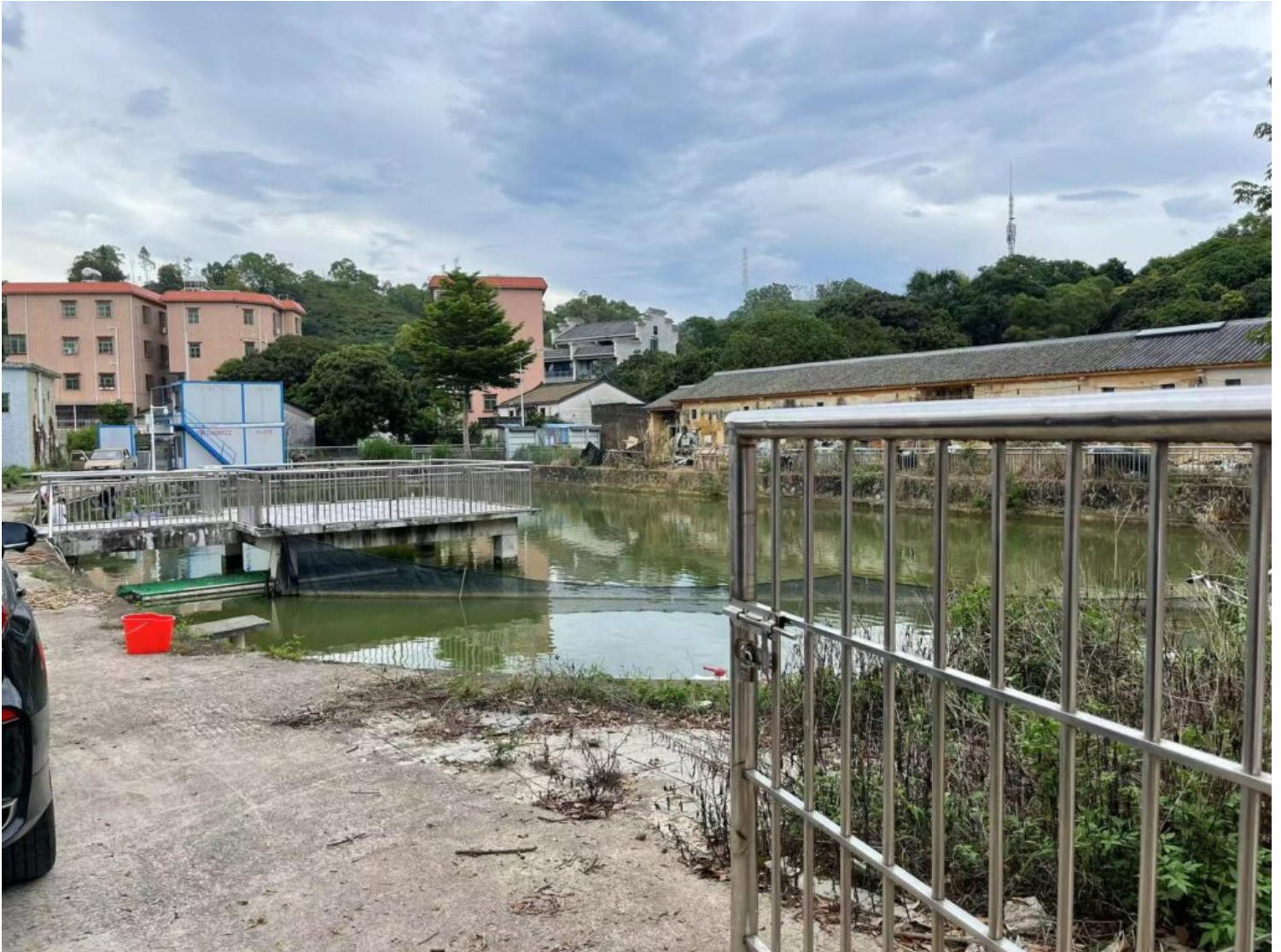
The pond before construction © Zhu Xiaodi
