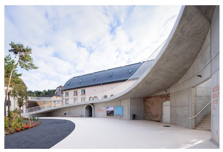
An undulating poured-in-place concrete surface alludes to glass production while it merges the buildings. The surface functions as roof, ceiling and wall, connecting the buildings' ground floors to shape a public plaza. New functions are sensitively introduced under and over this surface, including offices, workshop areas, a cafe and a restaurant.
