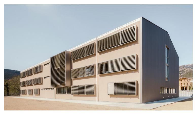
A wooden panel prefabricated system, and CLT (cross laminated timber) was used for both structures, vertical and horizontal, playing an important part in the way the project has been conceived.
