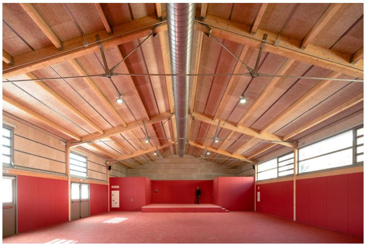
The CLT structural panels are coated when necessary (due to thermic, acoustic, or fire protection reasons) and remain uncovered when possible, as can be seen in the main hall and part of the roof's interior finishes, where the wood plays the leading role.
