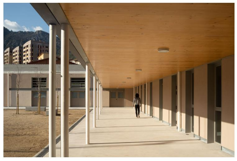
This system is widely known as reducing the structure and facades' environmental impact. Every cubic meter constructed with wood, implies a  $CO_2$  emission reduction of two tones. In addition, the water waste is near zero. The massive wooden enclosures contribute to the hygroscopic environmental regulation and the users' comfort. This improves the users' academic achievements, and makes the spaces more pleasant for them.
