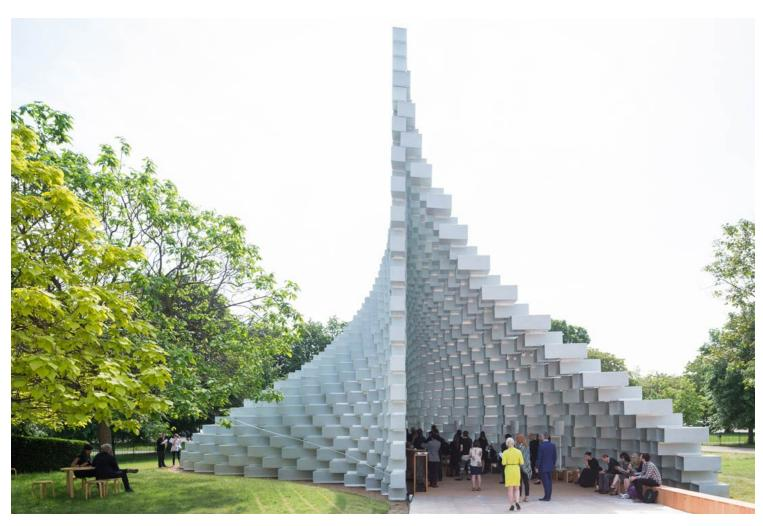
The unzipped wall creates a cave-like canyon, lit through the fiberglass frames and the gaps between the shifted boxes as well as through the translucent resin of the fiberglass. As a result the shifting overlaps as well as the movement and presence of people outside, create a lively play of light and shadow on the cave walls within.
