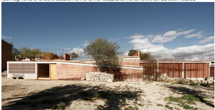
Next to a square, on the land of two abandoned vegetable gardens, the new building was designed: a small cultural facility with polyvalent uses and spaces. The construction, using local materials, provided the new topography to resolve the one-floor difference in level between the square and the gardens.
