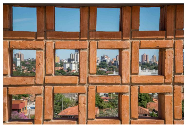
Fundamental elements of the design include the lattice wall on the west side (main façade) and cross ventilation in the building. There is a clear intent to control sun exposure. In addition to the lattice wall, made from red brick (a traditional material with strong roots in the country), which filters excessive sunlight, the spaces are well ventilated with big balconies and connections to the exterior.
