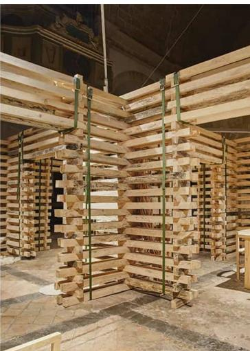
To build this structure, 950 slats of  $8 \times 4 \times 210$  cm were used, separated by 950 slats of  $8 \times 4 \times 30$  cm, held together by 84 straps. This system allows for the subsequent disassembly and storage of the wood to continue its drying process so it can be used to build furniture for the next Pollença Craft
