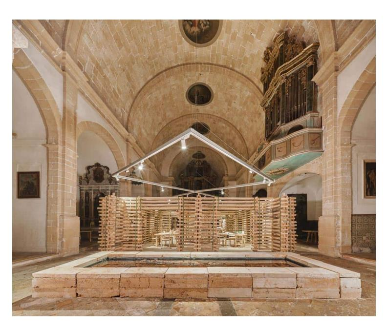
The third scene is a pine wood dryer built using slats sawn directly from the tree trunks. A total of 13 cubic meters of pine were used to construct 12 pillars using 2.1-meter slats (2.1 meters is the size used by Mallorca foresters, to fit the width of the trucks that transport the logs to the sawmills).
