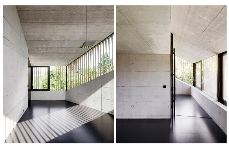
By milling the edges, the cross sections of the slats were modulated in correspondence with the window strip so that requirements of sight and sun protection were fulfilled, and various, flowing levels of transparency could be set.
