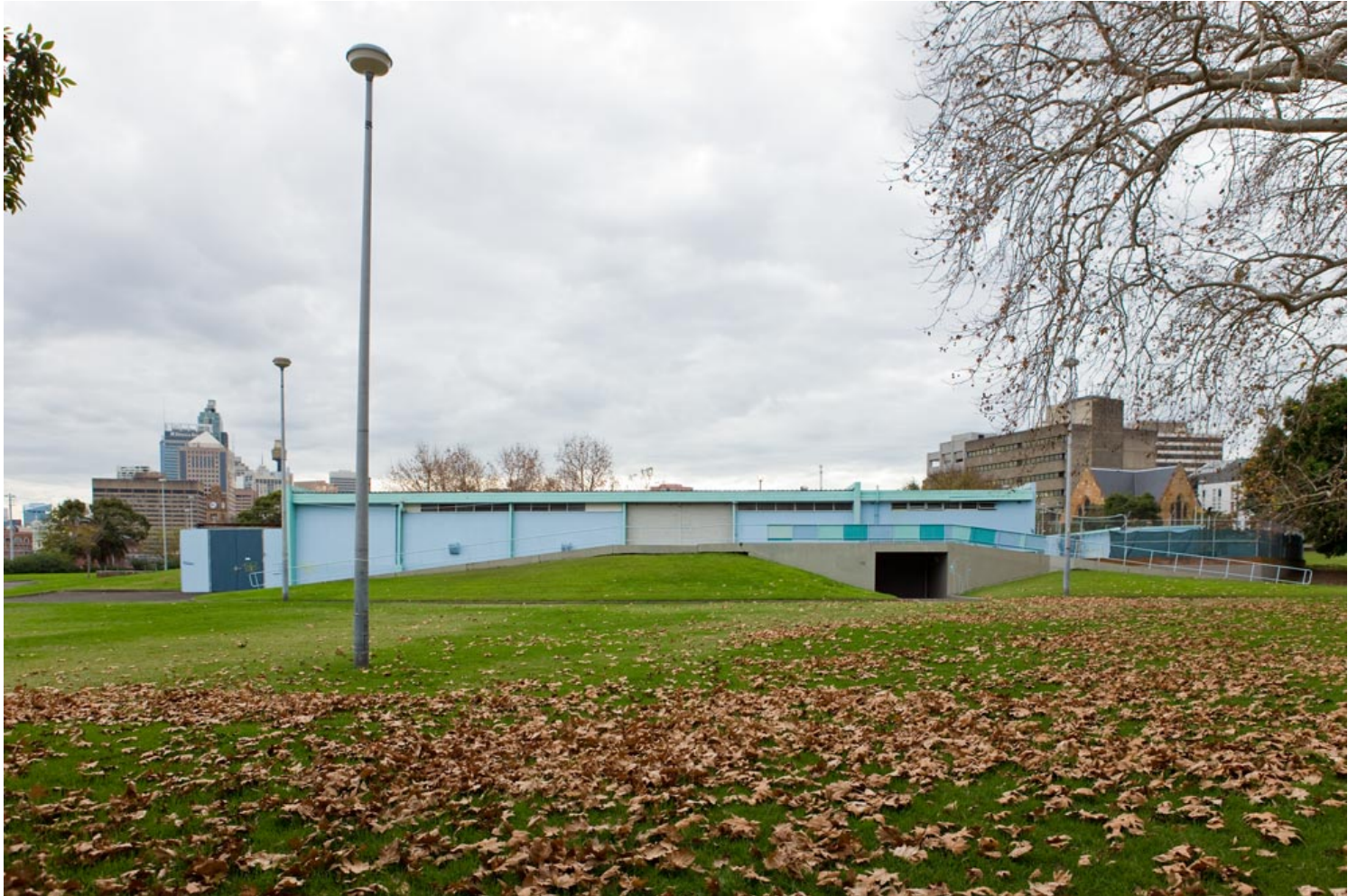
The pool prior to the upgrade.
