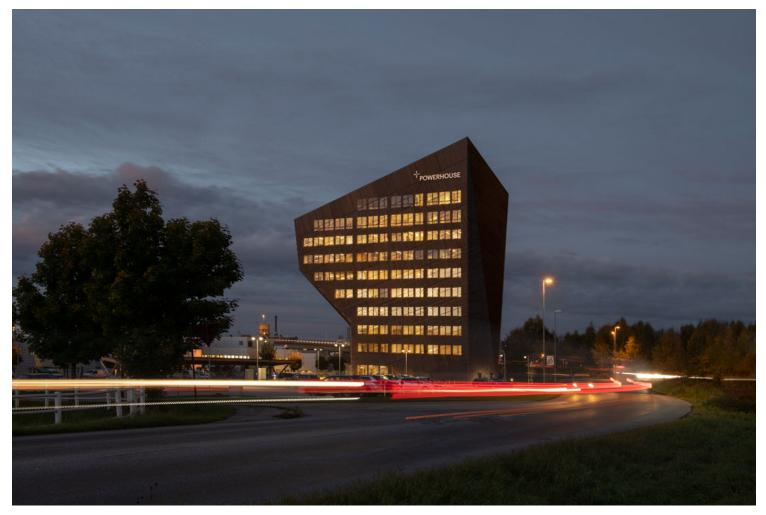
To the west, northwest and northeast, the building is clad with wooden balusters providing natural shading on the most sun-exposed façade. Behind the wooden balusters the building is covered with
