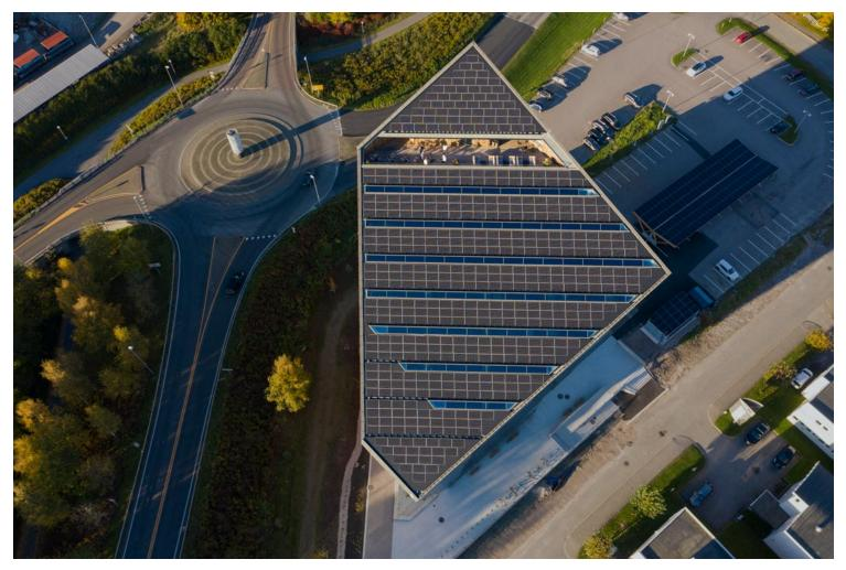
Powerhouse Telemark also utilizes a series of low-tech solutions to ensure that tenant comfort is prioritized, allowing the office building to be used to its full potential. The building's gently skewed west-facing and southeast-facing façades allow for a maximum of daylight and shading while also
