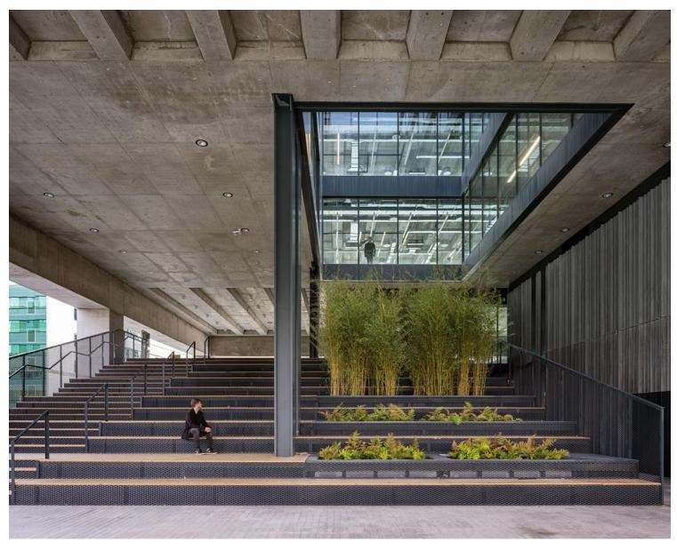
The definition of a perimeter structural line in coordination with the façade and the use of posttensioned slabs allows for a functional scheme of free plan in the work areas, providing versatility in terms of operations.
