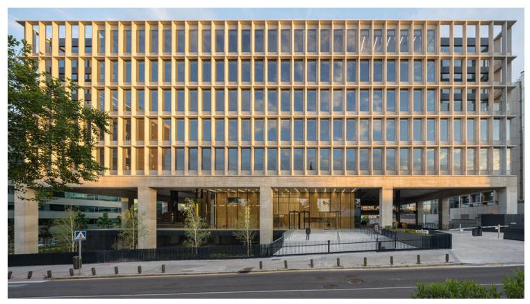
A prefabricated modular façade is defined by elements that adapt to the different climatic and lighting conditions. To the north, the opaque section of the façade is expanded to reduce costs and energy losses; to the south, the envelope is set back, creating a green strip for sun protection; on the east-west façades, the prefabricated concrete mullions are inclined to increase the shaded area.
