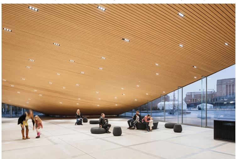
Oodi has been built using local materials and with local climate conditions in mind. The wooden façade is made from pre-fabricated elements. 33-millimeter-thick Finnish high-quality spruce has been used for the cladding. A specific grading and quality control system was developed for the timber, the sawing and the treatment of the slats. The complex curved geometry was designed and
