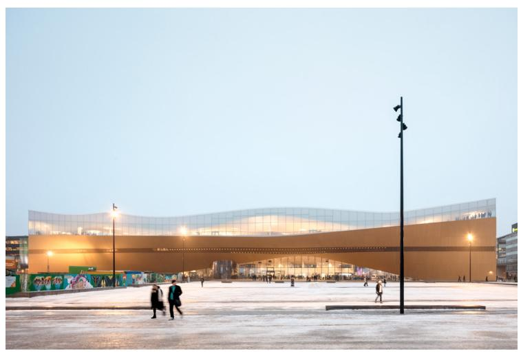
Oodi has been built using local materials and with local climate conditions in mind. The timber façade is clad with 33-millimeter-thick Finnish spruce planks that conform to the sweeping curve that extends the building outwards to create a canopy above the Kansalaistori square, blending the interior and exterior spaces and creating shelter for public events in front of the library.
