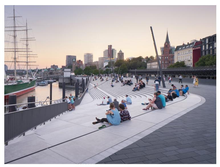
The linear structure is 8.60 m above sea level in its eastern section and 8.90 m above sea level in its western section to protect the city from maximum winter storm surges and extreme high tides.
