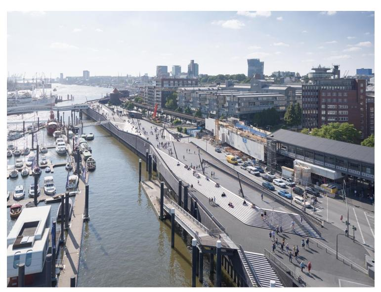
In the aftermath of storm surge floods in February 1962 that caused 315 fatalities and destroyed the homes of 60,000 residents, between 1964 and 1968 Hamburg developed a barrier on the banks of the Elbe at Niederhafen to protect the city against floods up to a height of 7.20 m above sea level.
