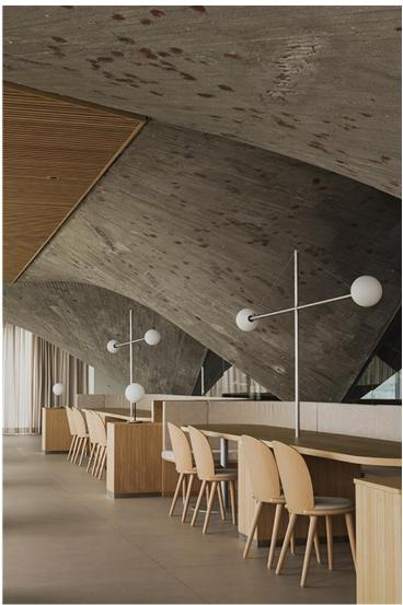
The square morphology of this volume is the result of the addition of 4 triangles that regularize and complete the paraboloids of the original building. Thus giving all the protagonism towards the interior to the rawness of these concrete paraboloids.
