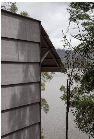
The house is entirely built in timber; only the façade is covered by thin fire-resistant fiber cement sheets. The footings are pinned to the underlying sandstone bedrock, avoiding the need for heavy
