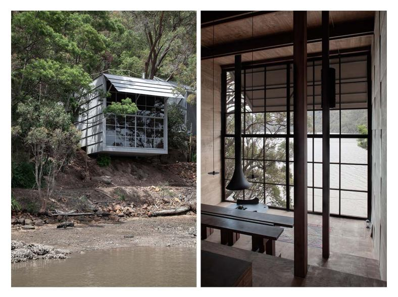
Marra Marra Shack is built using timber pillars made out of repurposed 200-year-old electrical posts used by the British, giving a new life to the Ironbark timber (*Eucalyptus crebra*). Spotted Gum timer (*Corymbia maculata*) growing in the Darug region is used for the beams of the ceiling and floor. The details and furniture are made of repurposed Turpentine timber (*Syncarpia glomulifera*) from the old jetty built by the settlers on the banks of the creek.
