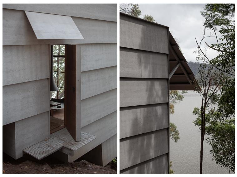
The house is entirely built in timber; only the façade is covered by thin fire-resistant fiber cement sheets. The footings are pinned to the underlying sandstone bedrock, avoiding the need for heavy
