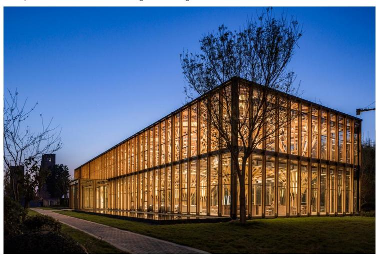
The cost-effective timber materials that we were able to purchase were square logs 3m, 4m or 6m long, with a cross-section 200mm wide. To build a large solid space and maximize its possible uses, several square timber pillars were combined together to form a "clustered column", instead of using
