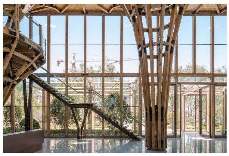
Considering various practical factors, we laid tiles on the ground floor by using cement mortar. However, all other constructing components shaping the space were connected by bolts. All of them can be completely dismounted, stored, moved and reused for other projects, making the building thoroughly reversible.
