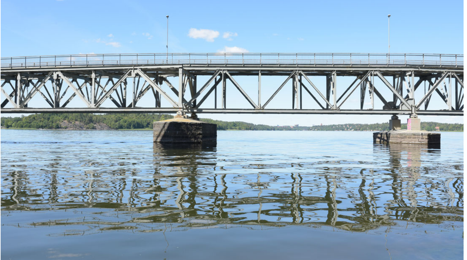
View of the structure of Gamla Lidingöbron (looking West).
