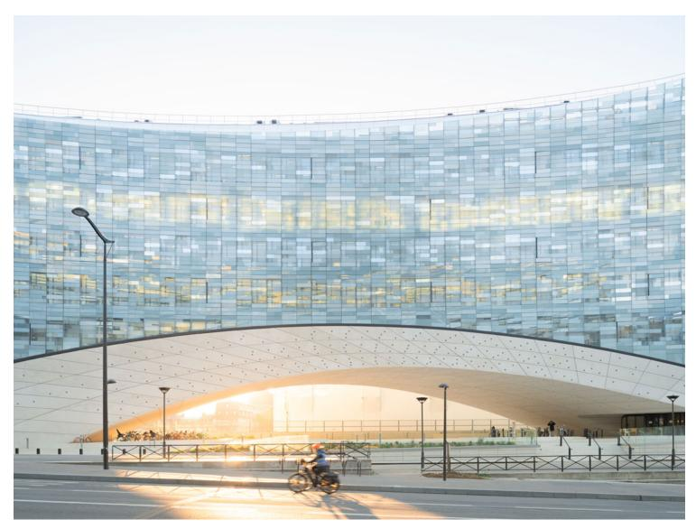
The materiality of the plaza is dominated by concrete with clear references to the building's urban context. The concrete environment creates a sense of continuity and consistency, as if parts of the ground were gently peeled back and fused into the arching roof soaring above the plaza. Cast in insitu concrete, the arch above the plaza is carefully hand-treated to create a textured finish.
