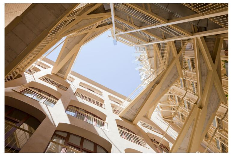
Although the heritage regulations allowed us to gut the entire building except the facades, the original structure of the building was preserved. The roof needed replacement, but the rest of the floors, walls and foundations were reinforced. Once the reinforcement was completed, the surplus of available loads was used to make the roof accessible and place a one-meter deep collective pool on top of the middle loadbearing wall.
