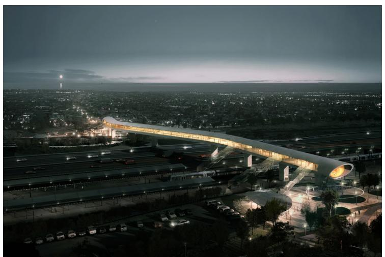
The main element of the design is a bridge combining Denmark's most trafficked freeway with the existing local Copenhagen train line and the planned double-tracked rail line for high-speed trains.
