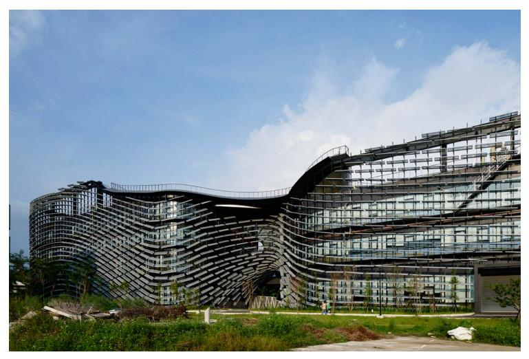
The fins are made of expanded aluminum sheet, creating a light-weight impression of the façade while allowing exterior views from the interior to some extent.
