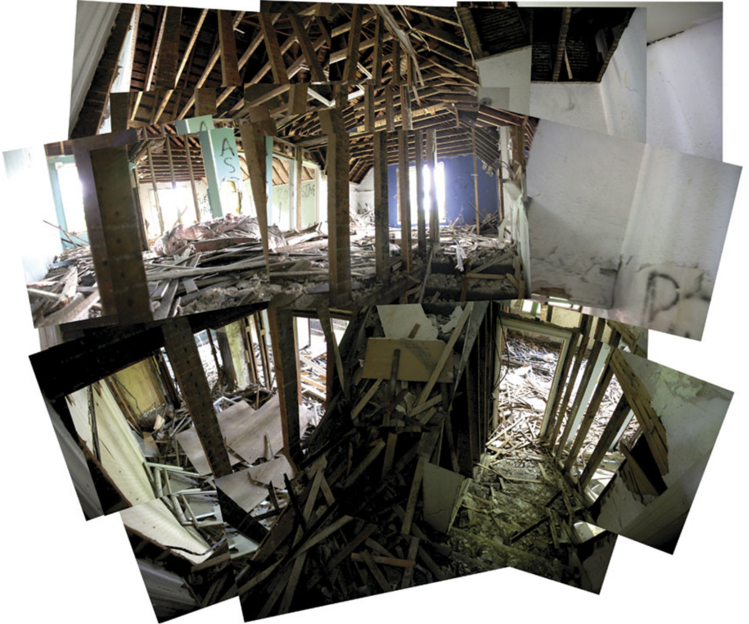
Interior demolition collage
