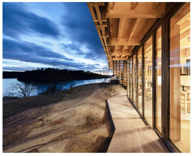
A prefabricated timber structure is placed on the concrete floors and, finally, a lightweight wooden structure covers the cabin to filter the light and direct the views. The wood structure has a depth that creates a play of shadows throughout the day and a calm atmosphere that resembles the feeling of sitting under a tree.
