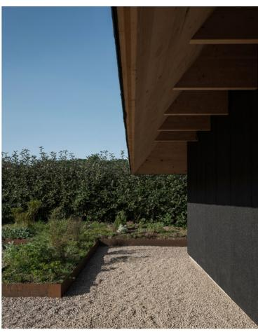
Carried by the cinderblock wall, the free-spanning glulam beams and the 16 skylights create a flexible space that can be configured to the shifting needs of its owners.
