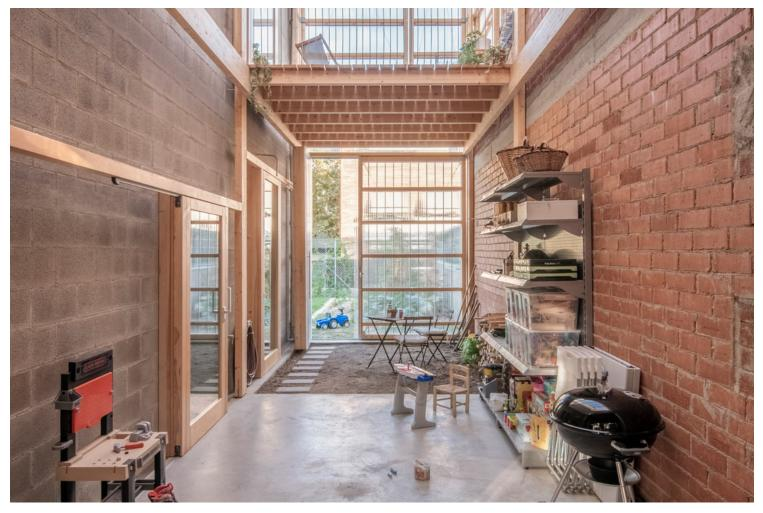
This intermediate space is resolved using lightweight construction (transparency, absorption, fast response), whereas the interior spaces are based on wet construction (thermal inertia, stability, slow response). The interior enclosures and the staircase are also lightweight, facilitating future modifications, unifying the spatial perception of the whole and making the surfaces in contact with users friendlier to the touch.
