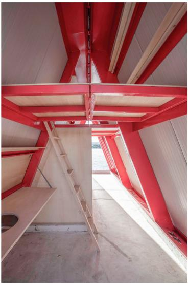
The unit is composed of two main parts: the upper structure that includes all the fixed furniture folded and implemented, and a floating pontoon made of concrete. The idea of a foldable unit which comes fully equipped is the result of research displaying that earthquake victims generally spend at least one year in temporary housing after the disaster.
