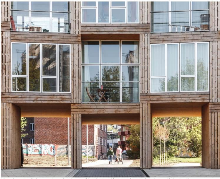
The characteristic checkered pattern of Dortheavej is based on a singular prefab structure. Conceived as a porous wall, the building gently curves in the center, creating space for a public plaza towards the street on the south side and an intimate green courtyard towards the north. On the street level, the building opens up to allow the residents and general public to pass seamlessly into the courtyard.
