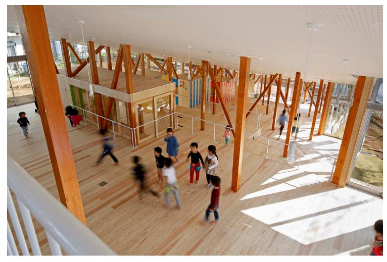
Utilizing large sliding window frames along the northern and southern faces, along with the space created by the slope, ventilation is created as a breeze draws in from the south of the structure, passes through the forest-like interior pillars making its way upwards before finally blowing out across the terrace on the northern side.
