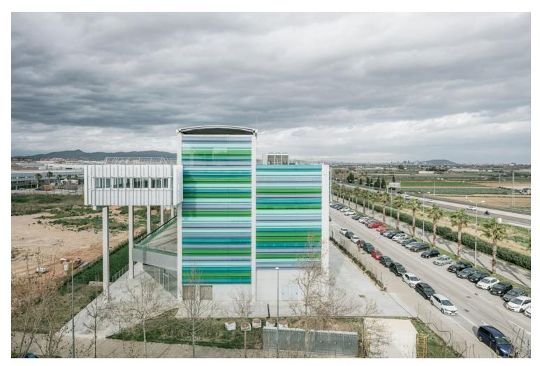
The building is oriented towards the C-32 highway. A double façade of perforated sheet metal evokes the chromatic patterns of the orchards that surround the building.
