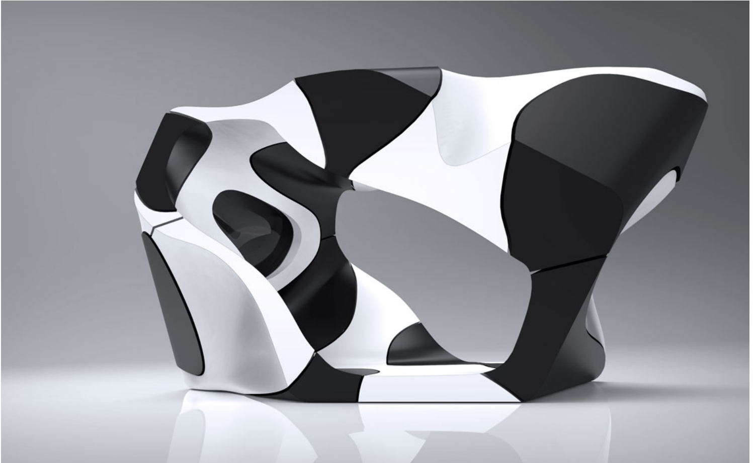
Fig. 03: The Plasticity Pavilion is a foam and fiberglass construction composed of large, nested elements.
