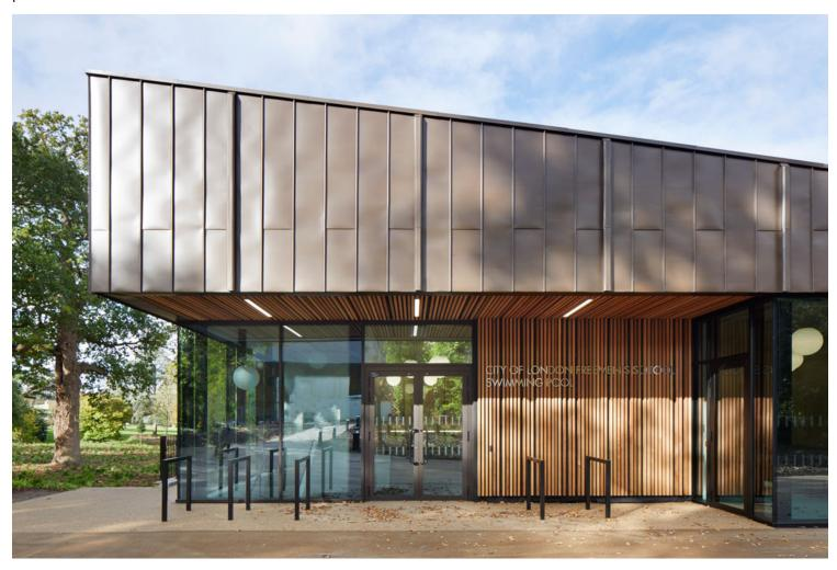
The all-timber construction also has a number of advantages in dealing with the challenges of a pool environment: it is resilient, a thermal insulator and corrosion resistant. On site, the erection of
