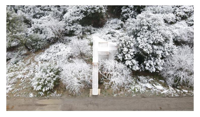
The CLT core rests on four glulam timber columns measuring 30 x 30 cm. The bridges are made from homemade glue laminated timber, the longest of which spans approximately 12 meters. These components were all individually made and then assembled using a crane in a highly intricate installation sequence. The CLT structure is protected by two layers of natural cork panels, providing thermal and acoustic insulation.
