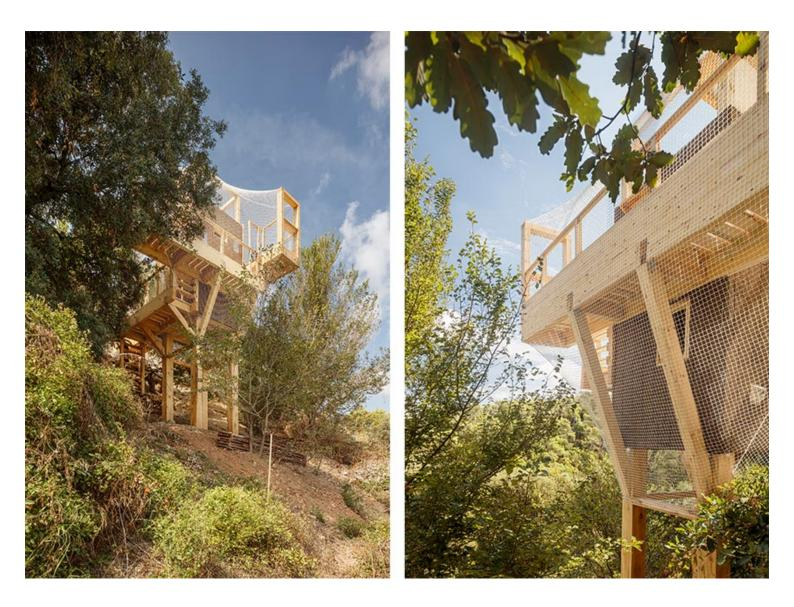
The surrounding net, which takes influence from a hunter's nest, was designed digitally and then woven by hand. The net is intended to better camouflage the construction by allowing plants to grow across it, thus further merging the structure with the forest in order to hide it from the surrounding wildlife.
