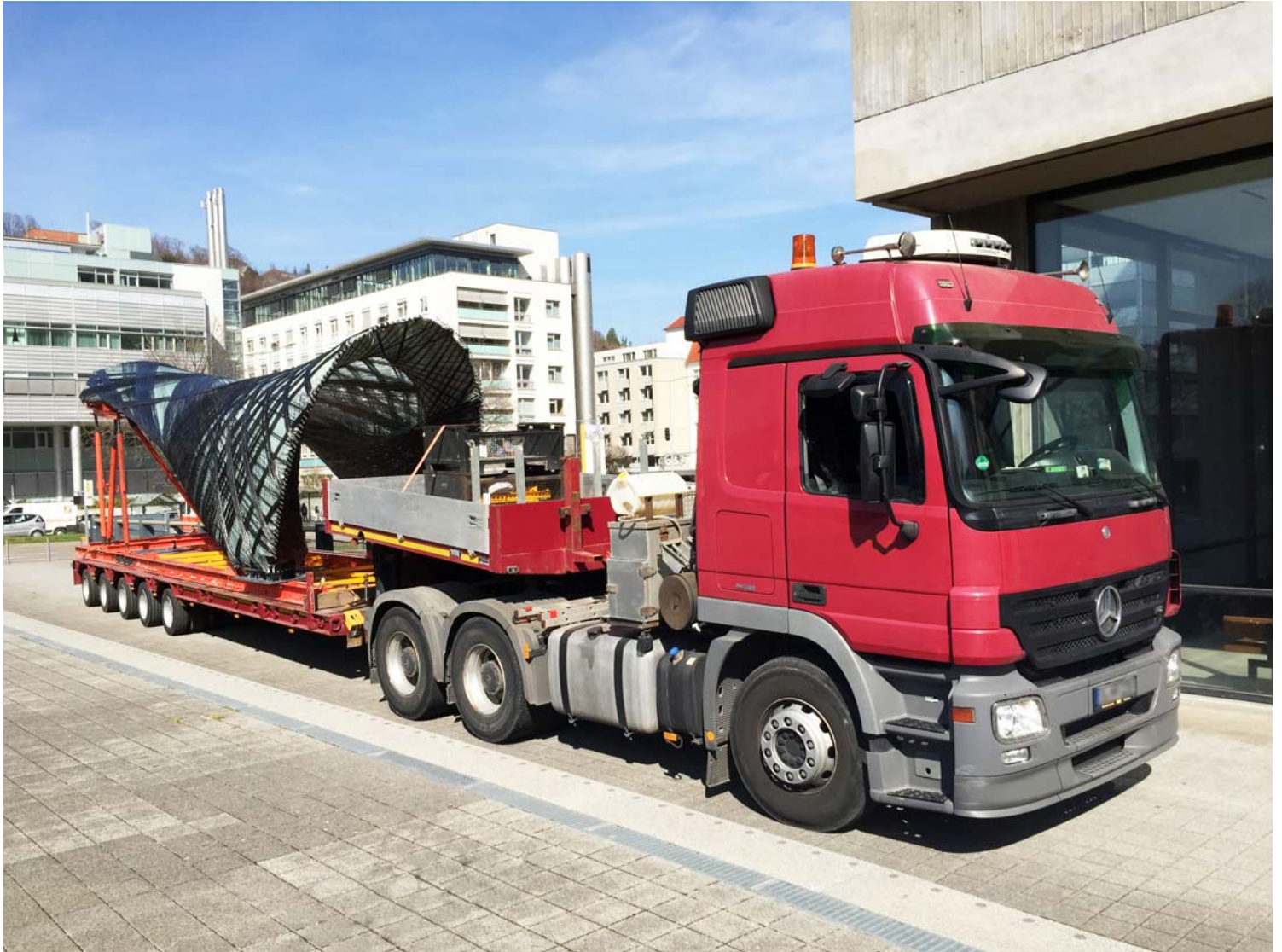
Transport of long span fiber composite structure to site
