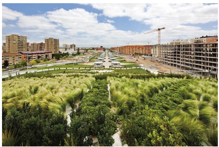
The project began with the knowledge that Logroño has a large underground irrigation system fed by the Ebro River, a condition that made it possible to create of a large green space for citizens. The green roof over the infrastructure serves as thermal insulation for the stations, which not only saves
