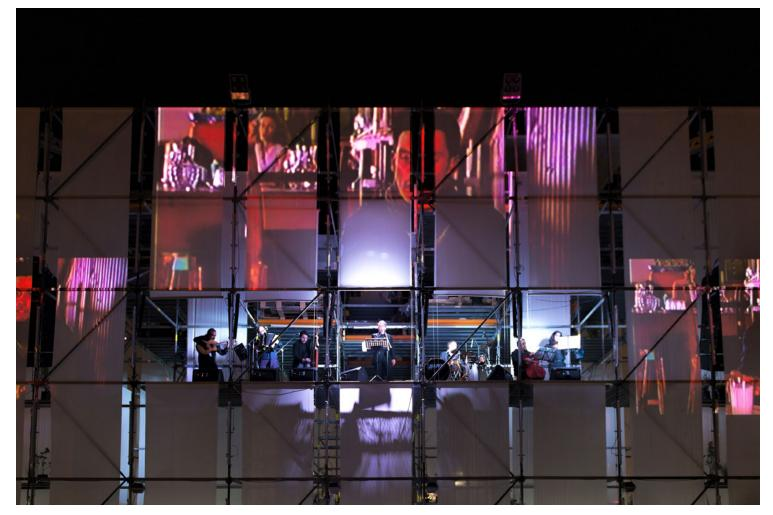
A light construction composed of a multidirectional scaffolding framework covered by polyester fabric strips that lends different degrees of transparency to the volume.
