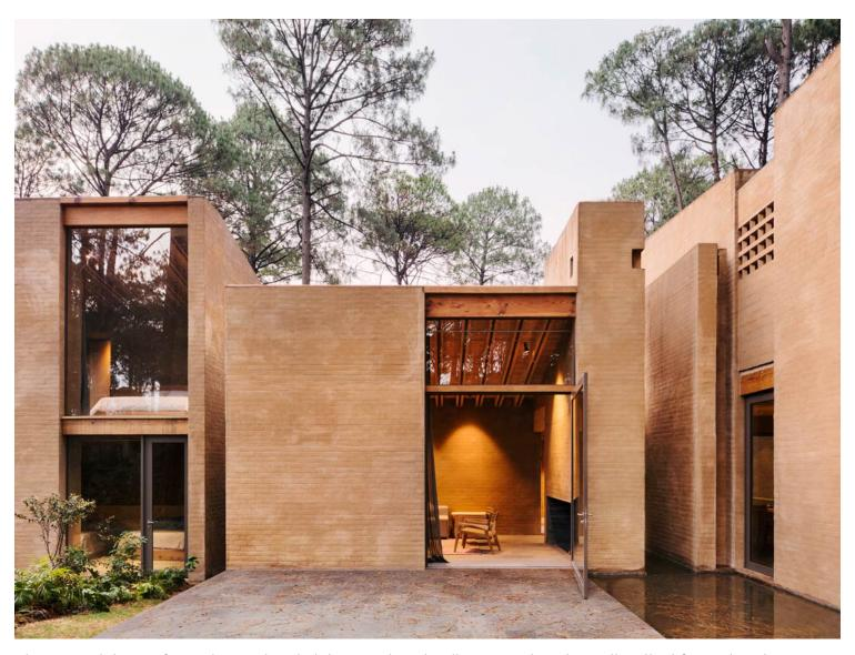
The materials are from the region: brick, wood and soil. By reusing the soil culled from the site to cover the walls, the five buildings have a warm, natural and terracotta colour finished.
