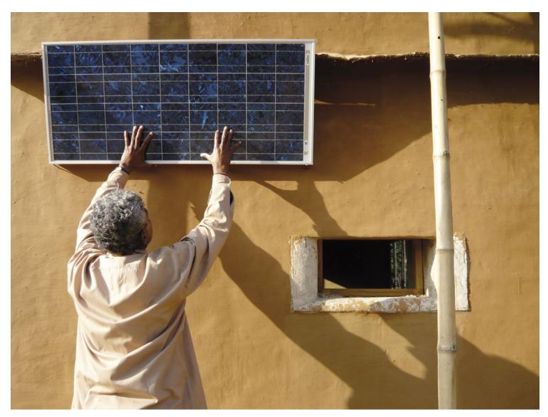
The building is an appropriate balance of high tech and low tech: very basic building methods are combined with modern, alternative energy power systems. Because the building is passively heated and cooled and optimizes natural light and ventilation, the relatively small solar panel and battery system provides all of the power the building requires.
