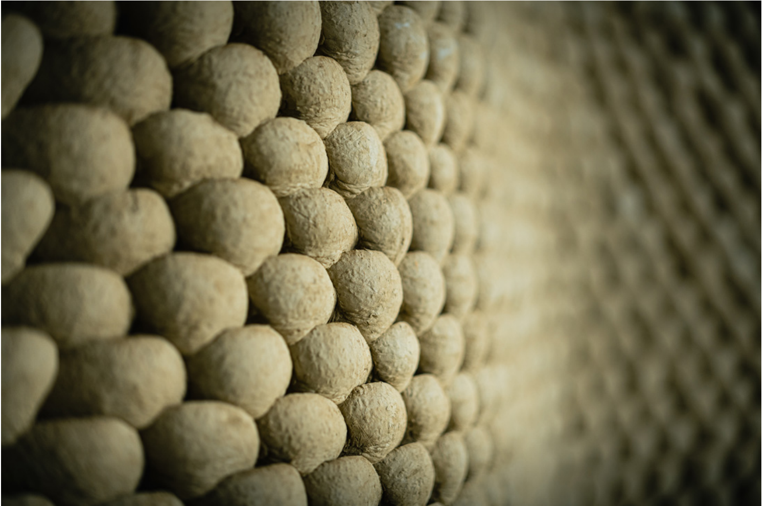
Clay Rotunda, detail view of the soft bond, 2020-2021 © Gramazio Kohler Research, ETH Zürich. Photo: Michael Lyrenmann
