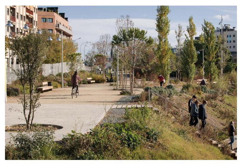
A sustainable drainage system was built to control and manage rainwater, collecting it in gravel ditches and green trenches. These systems give the water a laminar flow, channeling it to the retention biotopes until it evaporates or seeps into the ground. This prevents water from being discharged into the municipal sewage system, and manages it in a self-sufficient way.
