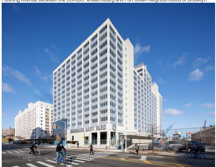
The building was rapidly constructed in 1942 as a 16-story reinforced concrete structure. The windowless lower 11 floors provided warehouse storage, while the upper floors served as offices for the Yard's Commandant and the US Navy's oversight of the North Atlantic Fleet during WWII. The building is a part of the National Register Brooklyn Navy Yard Historic District.
