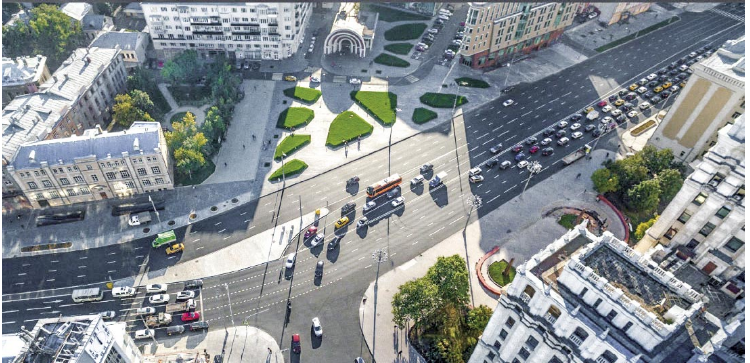
The square in front of the Krasnye Vorota metro station before and after reconstruction © Moscow Municipal Services Complex
