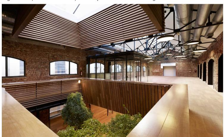
The intervention showcases the history of the factory building, revealing the original structure in steel and brick, combined with the newly executed finishes, mainly in oak, steel and glass.
