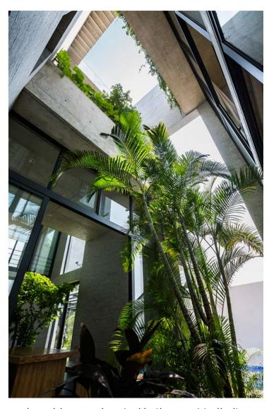
Service areas such as the kitchen, bathrooms, stairs and corridors are located in the west to limit heat radiation exposure towards frequently occupied areas. The vertical variation of spaces creates a lopsided pressure difference. Thus, when the surrounding houses are built, natural ventilation is maintained. Thanks to these passive strategies, the house always stays cool in the tropical climate. The air conditioning system is rarely used.
