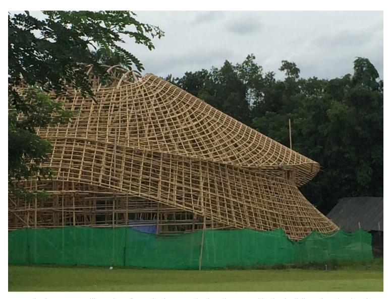
Panyaden's Sports Hall's carbon footprint is zero. The bamboo used in the building absorbed carbon to a much higher extent than what was emitted during treatment, transport and construction.
