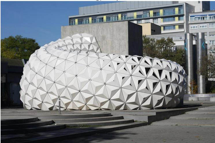
Collaborating materials scientists, architects, product designers, manufacturing technicians, and environmental experts were able to develop a new material for façade cladding which is thermoformable and made primarily (>90%) from renewable resources. Developed by project partner TECNARO within the framework of the research project ARBOBLEND®, a special type of bioplastic granules can be extruded into sheets which are further processable as needed: they can
