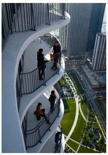
Early and close collaboration between architect and builder, as well as the use of contemporary digital tools, allowed the variation in the shape of the floor slabs to be achieved without increasing the building's construction timetable. The result is a high-rise tower particular to
