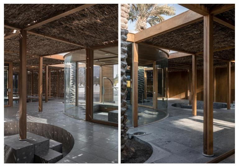
A tight grid of timber columns and beams is used on the site as both an organizing principle and a reference to the date palm plantations in the north of the island, irrigated by a complex network of water channels. The resulting building is a low single-story construction stretching the entire boundary of the site. Only the palm trees pierce through the horizontal ceiling to become the expression of the building.
