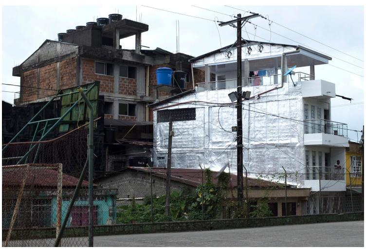
This self-adhesive asphalt is easy to install and is an excellent sealant that conforms to any surface. Made with elastomeric polymers and fiberglass, this product is quite elastic, flexible and durable, resistant to traction and weathering, and it can withstand sudden changes in temperature and can keep the temperature of the exposed surfaces and inner spaces within comfortable limits.
