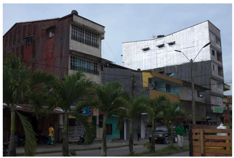
Within Quibdó, wood and bamboo cane have mostly been substituted by cement blocks and bricks, while palm leaves have been replaced by zinc roofs. Zinc or galvanized steel roofs, introduced into the city in the late 19thth century, were the first modern architectural element to be incorporated into local architecture. Wire screens for the doors and windows, which kept disease-spreading mosquitos out, also became an essential element of 'modern' constructions, adding a metallic shine.
